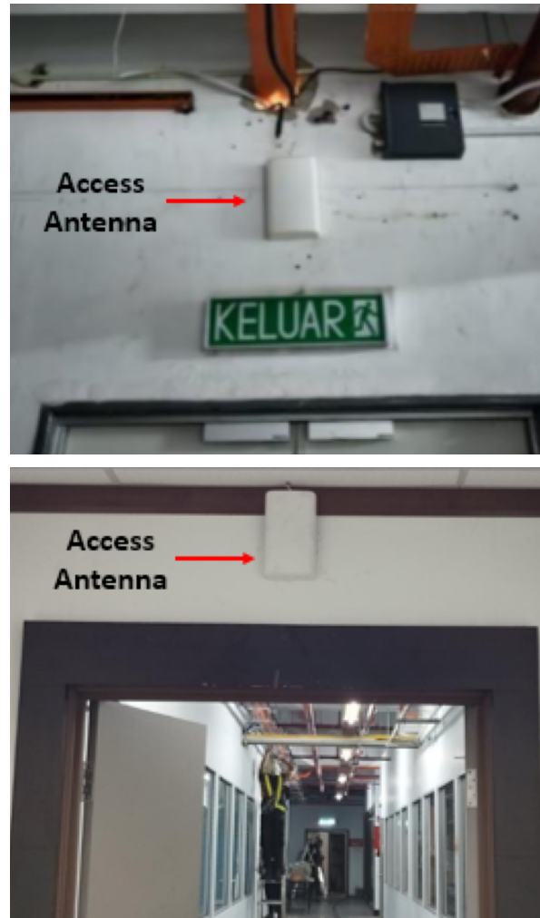
Figure 5: Access Antenna installed at Level 2 and Level 3
